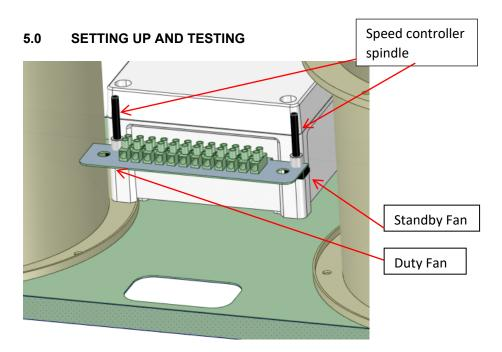
The duty and standby fans are each fitted with a speed control module. These are located adjacent to the fan and is adjusted using the black spindle which is mounted on either side of the terminal connection block as shown in the picture above. Do not bend the spindle.
