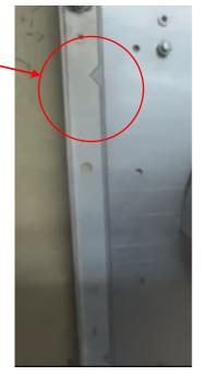
Note that the brackets are handed and the locating tags are in different positions to ensure the fitted to is fitted correctly.
